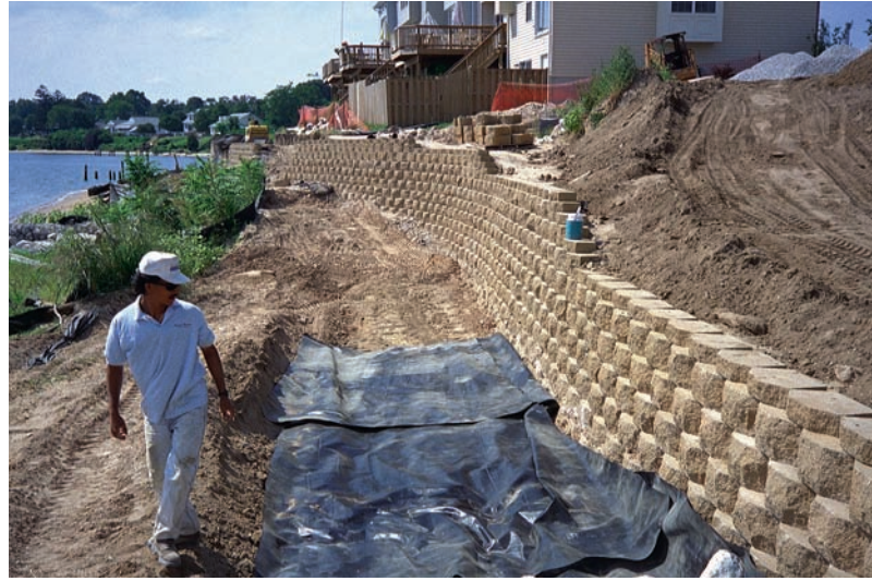
Installing the rip-rap at the base of wall
