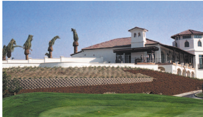
Combination of reinforced slopes and Keystone walls at clubhouse.
