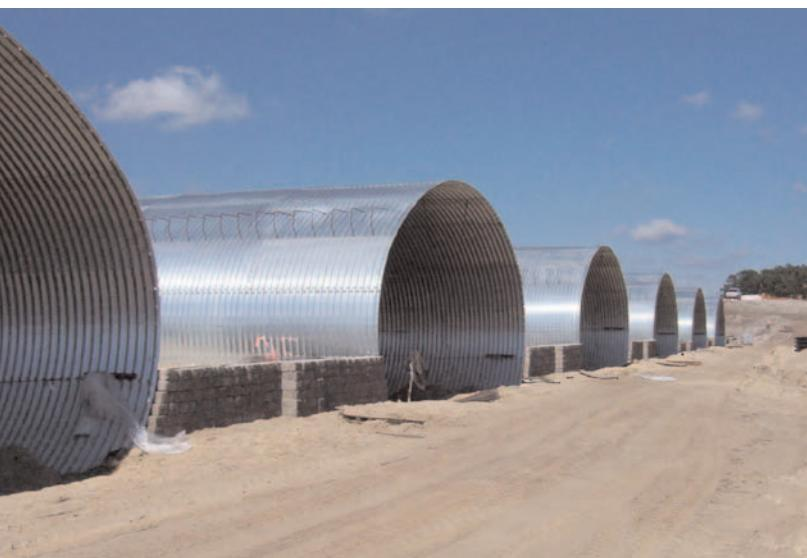
Products proposed a ten-barrel, horizontal-ellipse Super-Span system requiring only minimal subgrade remediation. Keystone Country Manor segmental retaining wall system headwalls then surrounded the CONTECH bridge structure. The Keystone Country Manor walls added the aesthetic appeal that was desired for this upscale planned-community, and their versatility offered the design and installation freedom necessary to complete this complex and extensive structure.
