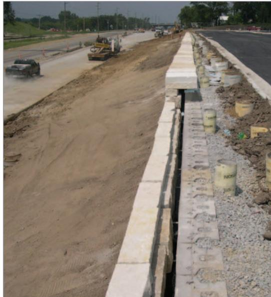
approximate dimensions of the limestone blocks were 12 inches high, by 30 to 36 inches wide, by 14 inches deep. The Keystone Compac wall was assembled in a near-vertical configuration to a maximum height of approximately 10 feet along the 465-foot length of the structure. Behind the Keystone wall, a four-inch perforated PVC drain-tile with sock was installed to assist with water flow through the crushed stone fill.
