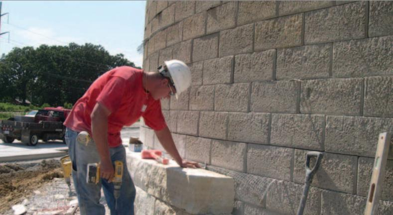
In order to flex, expand and contract as a cohesive system, the limestone veneer was dry stacked in front of the Keystone wall to which it was attached. The limestone veneer was attached to the Keystone Compac Straightface units with a Tapcon™ screw and a stainless steel, "z-shaped" strap system.
