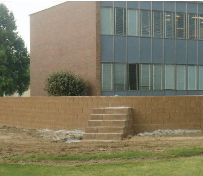
The unique design left a smaller area for wall installation crews to work within that came into effect when needing to get 100% compaction without pushing either one of the walls out. According to Contractor Jeremy Banken of Structures, even with the space constraint, installation did not require use of special equipment or change in method.
