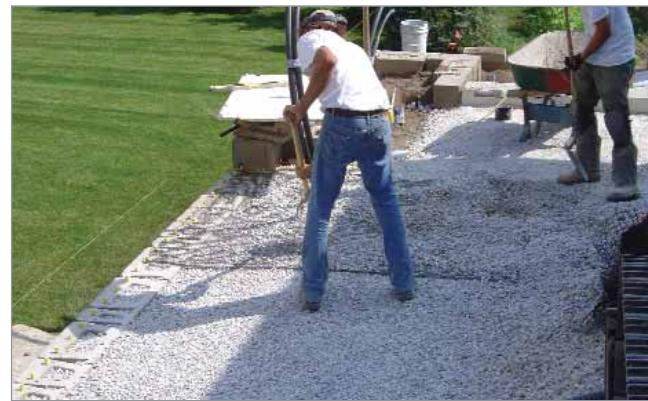
An underground drainage system that empties into the southwest corner of the backyard handles storm water runoff. The critical needs were to prevent water from backing-up into the lower level walkout and prevent surface water running into the pool. The underground network of collection pipes empty into a catch basin. The catch basin empties into a 10'x 10' French Drain. The French drain is located below the freezing line to an approximate depth of 14'. The area is backfilled with clear stone.
