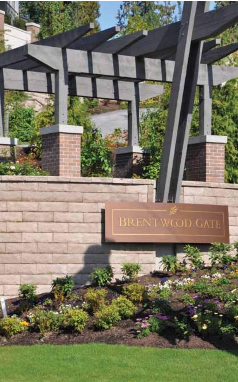
The project spans about 1200 feet and is approximately 30 feet high, making it one of the highest segmental retaining walls in the Vancouver area. About 30,000 square feet of 133Elite units were used for the upper tiers. A reinforced concrete wall forms the lowest tier.
