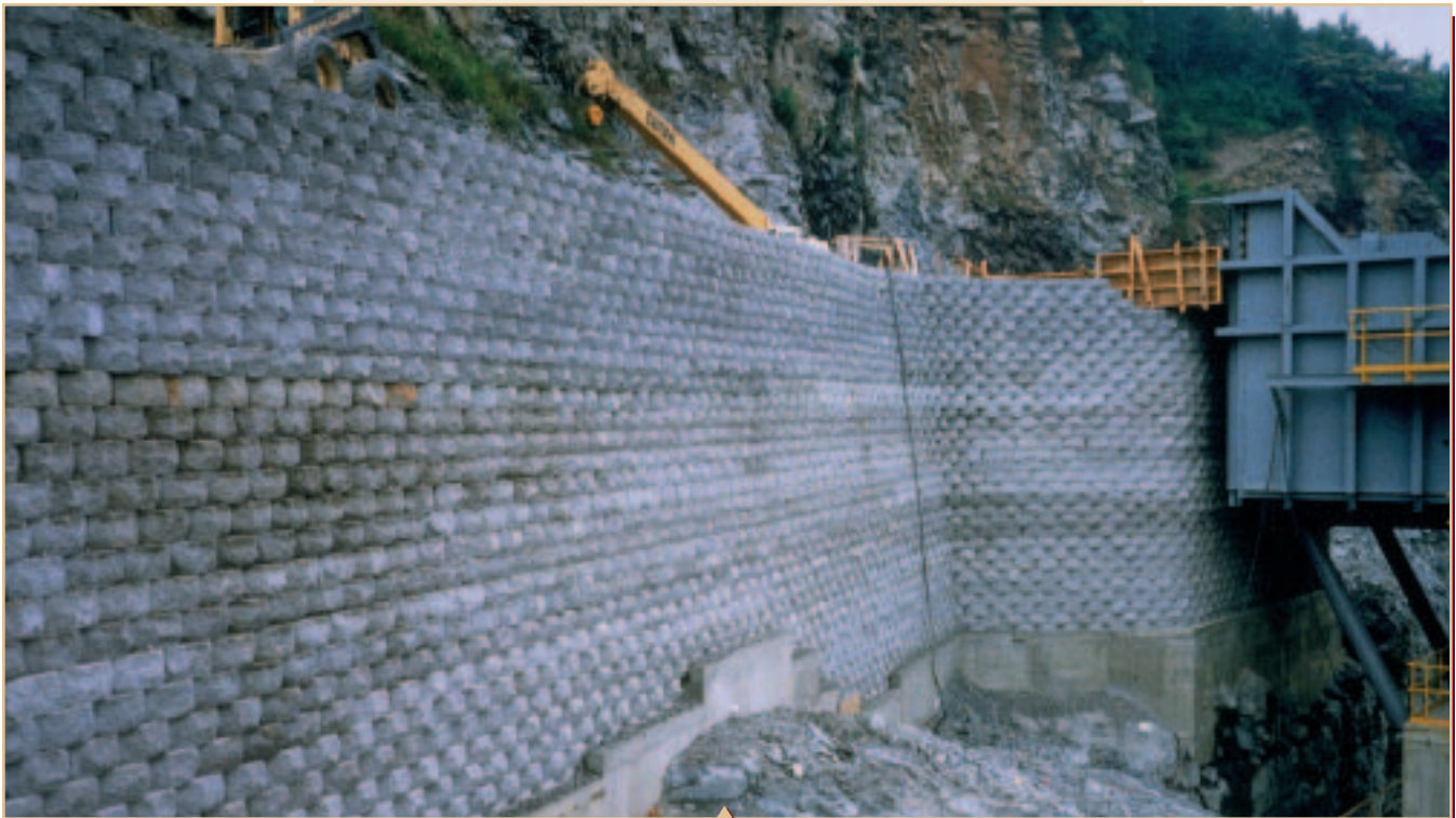
Keystone wall constructed on a reinforced concrete footing.
