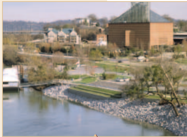
Retaining Wall Solution Protects Park Area
