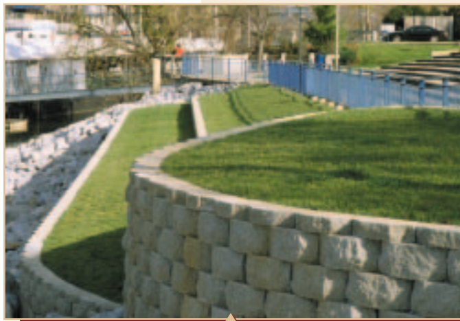
New Terrace wall protects amphitheater from erosion
